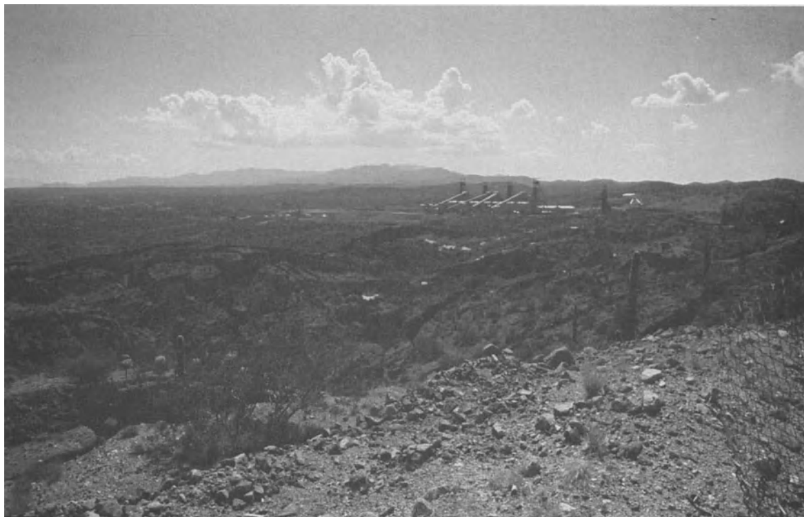
Fig. 3.5 San Manuel Mine, Arizona, is one of the few underground mines producing from porphyry copper deposits. The surface subsidence in the foreground results from the caving method used to mine the San Manuel ore body. Beyond the headframes lies the Kalamazoo ore body.
