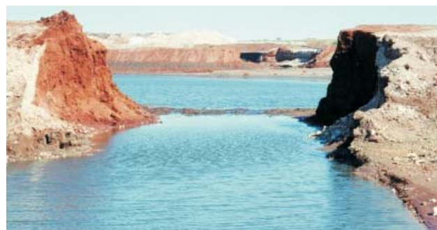
FIG 1 - A gateway to hell: the result of poor embankment design and operational planning for a tailings storage facility.
