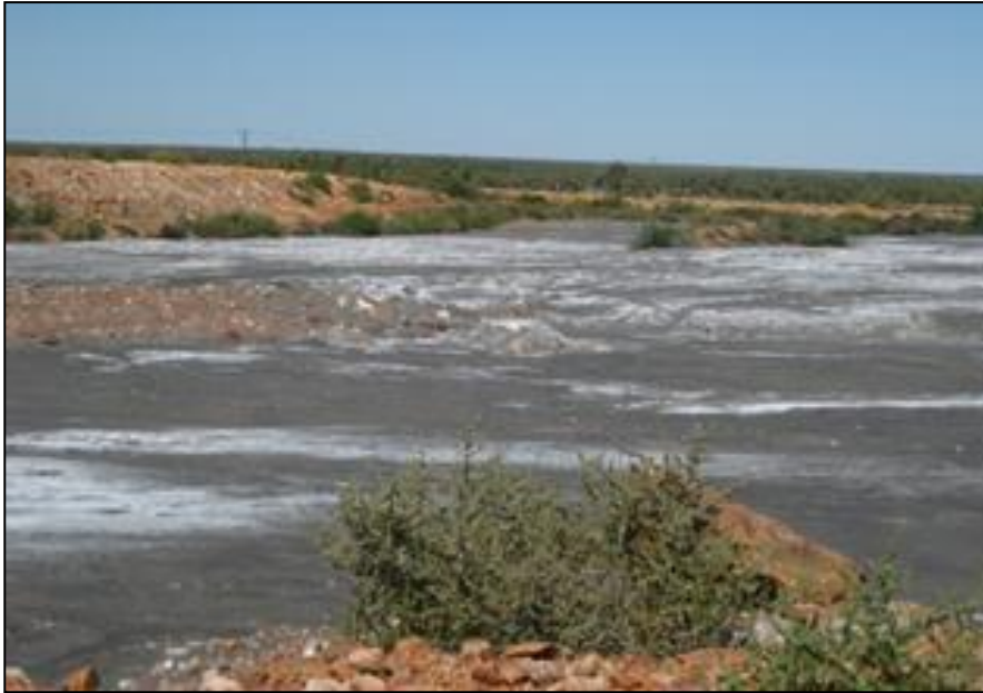
Figure 20-7: Salt Crust on TSF2
