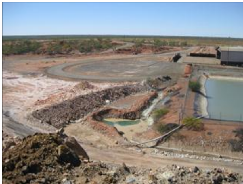
Figure 20-10: Drain/sump showing possible metal leaching
