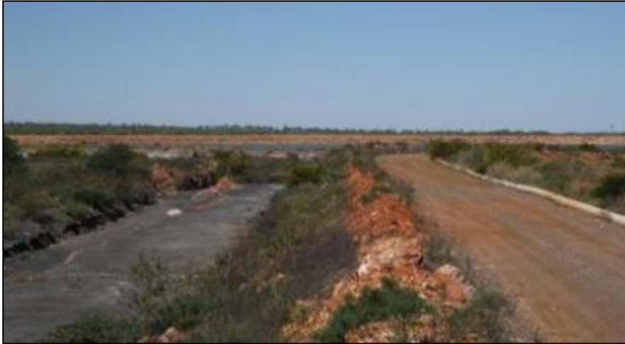
Figure 20-5: View of TSF2 looking north towards deposition point
