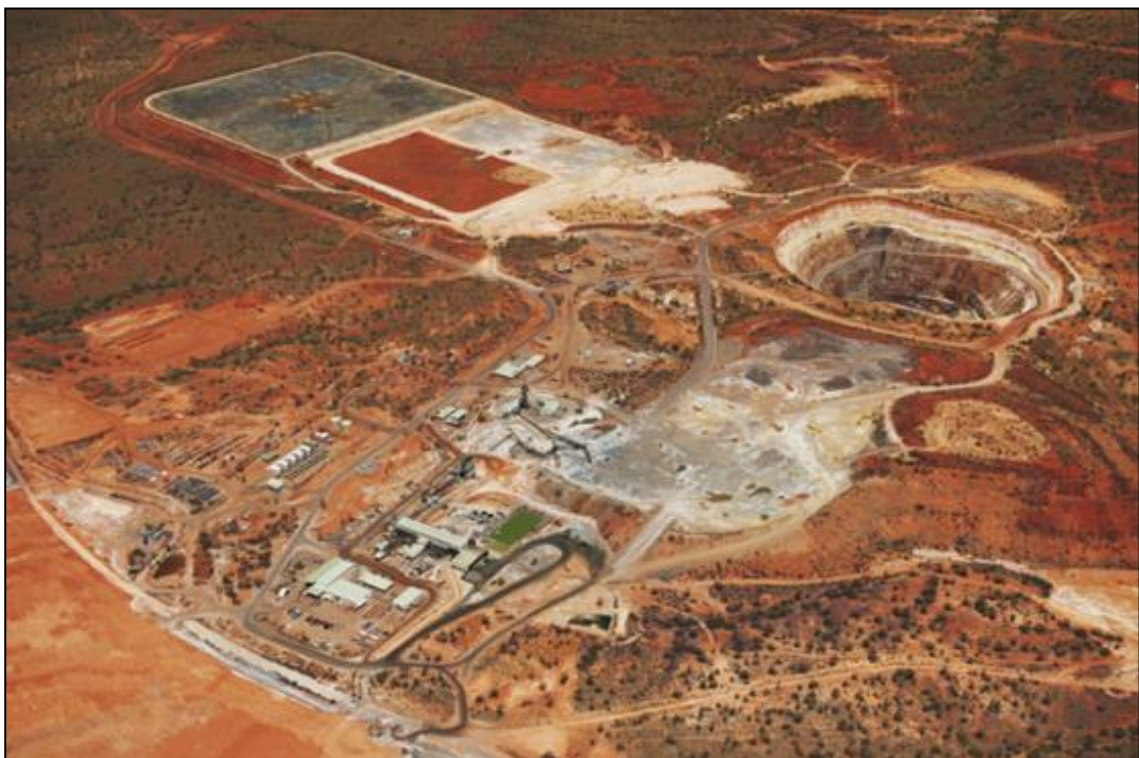
Figure 5-3: Osborne mine infrastructure
