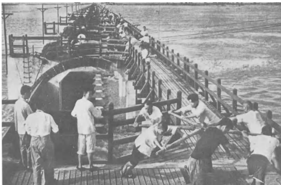
Plate 7.10. Adjustment of water flow through a weir at Tai Ping Kou flood detention basin on the Yangtze River, China (from R. Alley, 1956)
