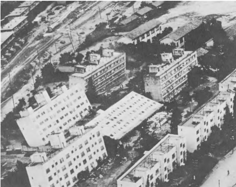
Plate 1.4. Liquefaction of saturated sands led to tilting of apartment buildings in Niigata in 1964 earthquake. (Courtesy of T. Mikumo)
