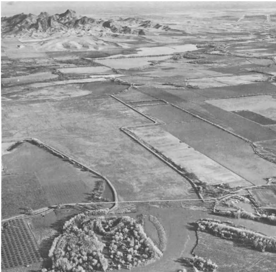
Plate 7.8a. In the foreground can be seen the Colusa by-pass weir in California. In the background to the east are the Sutter volcanic buttes. In the dry summer, the land used for storage is cultivated. (Courtesy of California Department of Water Resources)
