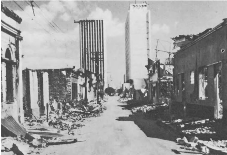
Plate 1.2. The great variation in damage in the Managua 1972 earthquake. The torquezal dwellings (space between vertical wood studs is a “pocket”, packed with mud and stone) collapsed (high intensity rating?) but the modern Banco de America building in the background stood with no substantial structural damage (low intensity rating?). (Courtesy of M. Sozen)
