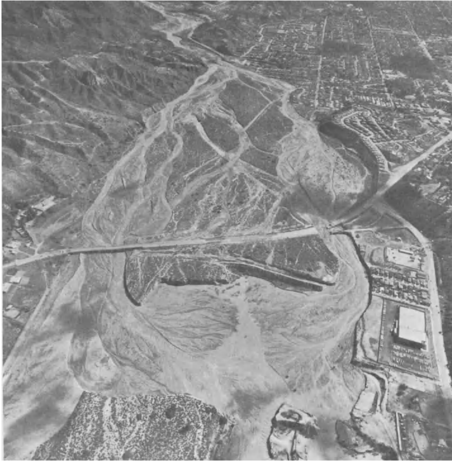
Plate 7.4. In Los Angeles County, California, February 1969, flood flows came roaring out of Big Tujunga Canyon, destroying Foothill Boulevard Bridge (upper bridge) and Wentworth Peace Bridge. (Courtesy of Los Angeles County Flood Control District)
