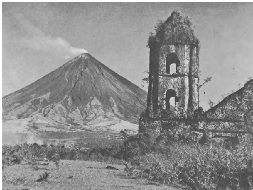
Plate 2.8. Church in Cagsaua, Philippines, buried to the top of the nave by a mudflow from Mayon Volcano (background) in 1814. It is reported that the people of the village had gathered in the church for refuge and all were killed
