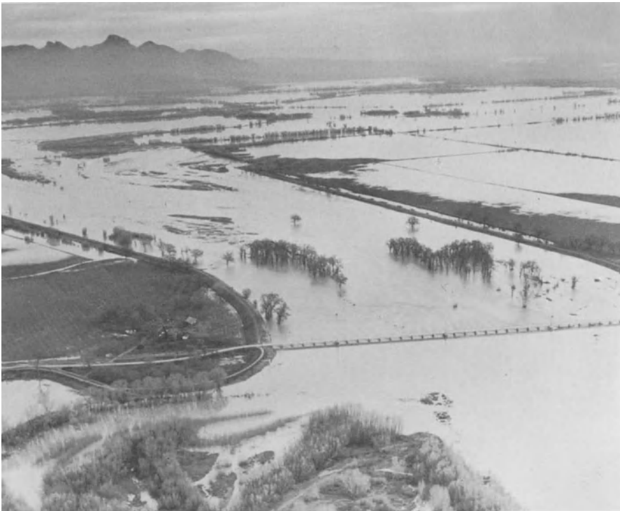
Plate 7.8b. A similar view of the Colusa by-pass weir to that above showing water passing over it into storage during high water on the Sacramento River. (Courtesy of California Department of Water Resources)
