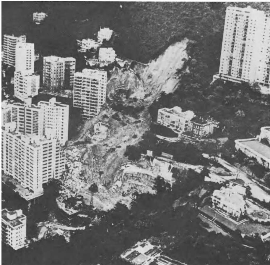
Plate 4.1. Hillside failure, Hong Kong. (Courtesy of Fugro, Inc., Long Beach)
