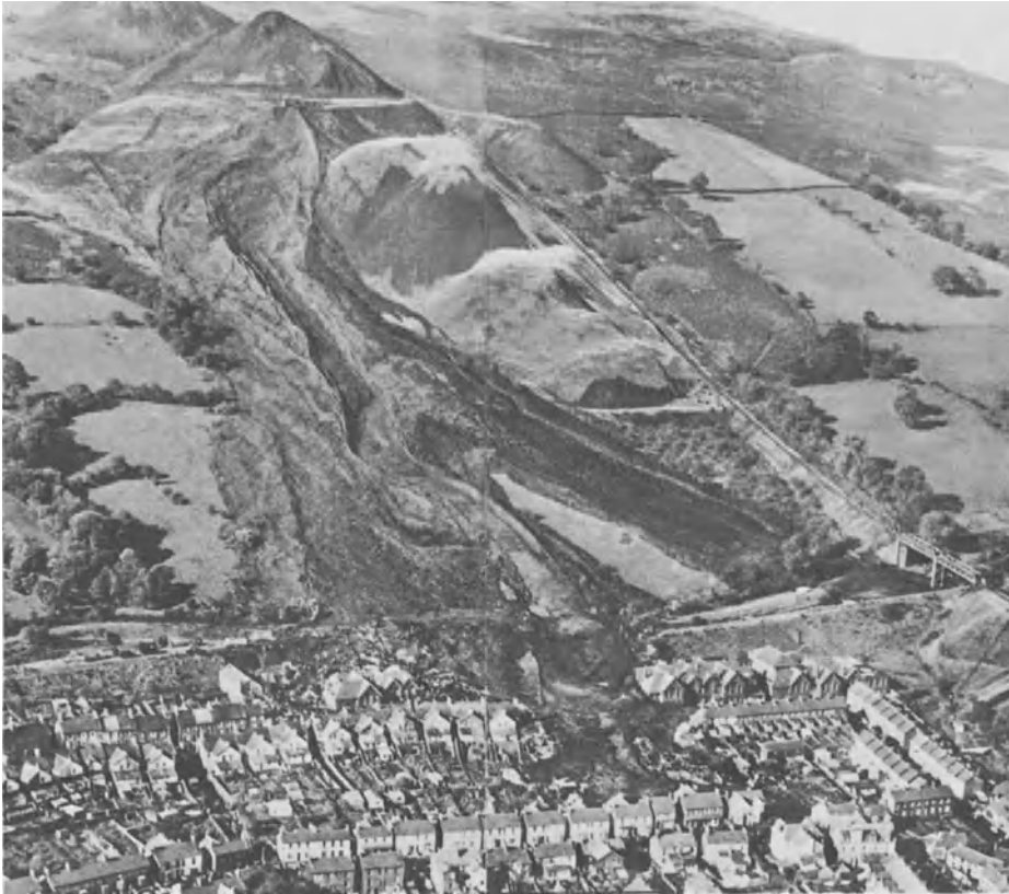
Plate 4.6. Failure of Tip No. 7, Aberfan, Wales. (Report of the Tribunal of Inquiry, HMSO)
