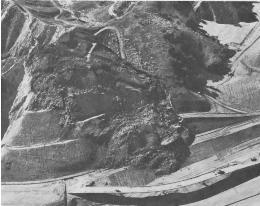
Plate 4.3. Landslide in cut slope during San Fernando earthquake of February 9, 1971. (Courtesy of State of Calif. Dept. of Public Works)
