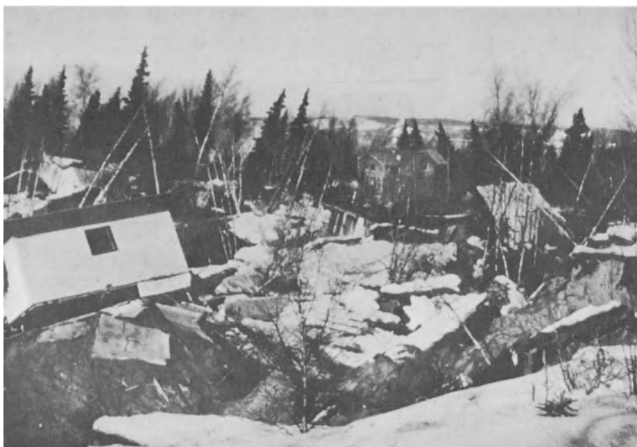
Plate 1.1. View of damaged houses due to great slide at Turnagain in 1964 Alaskan earthquake. Soft clay bluffs about 22 m high failed in the shaking. The slide extended 2,800 m along the coast-line and regressed inland 300 m. (Courtesy of USGS)
