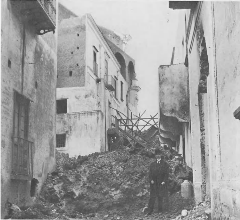
Plate 2.5. A lava flow in the streets of Bosco Trecase, during the eruption of Vesuvius in 1906. The thrust of the lava was not sufficient to cave in the masonry walls. (Photo by T.A. Jaggar)
