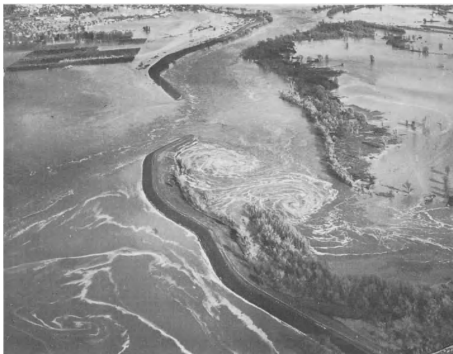
Plate 7.7. The breach of a levee on the Feather River, California near Yuba City, during the floods of December 1955. (Courtesy of California Department of Water Resources)
