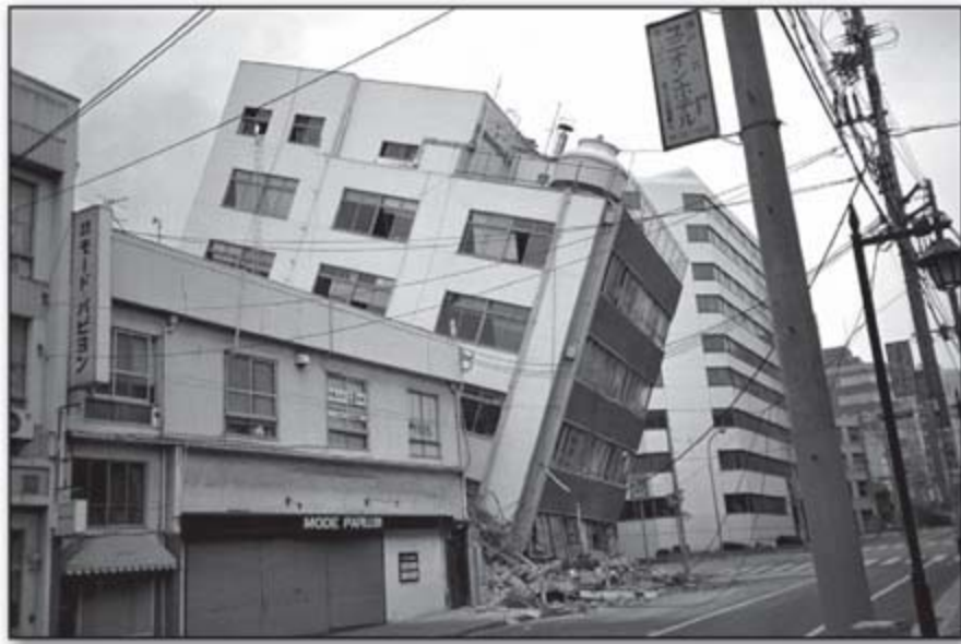
Building knocked off its foundation by the January 1995 earthquake in Kōbe, Japan. Dr. Roger Hutchison/NGDC
